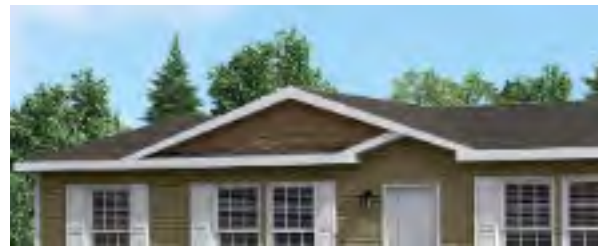
Shake Siding on Dormer above Continuous Eave
