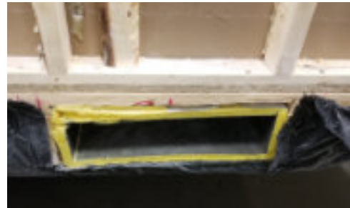
Fiberglass Heat Ducts w/ In Floor Cross over Heat Ducts
